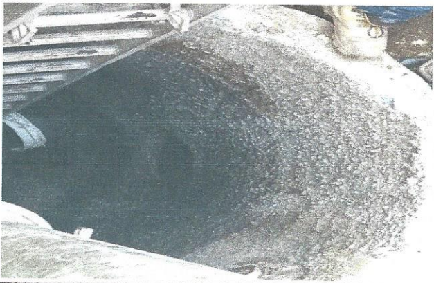
Lift Station prior to the application Alumiliner and Raven 405 Epoxy
