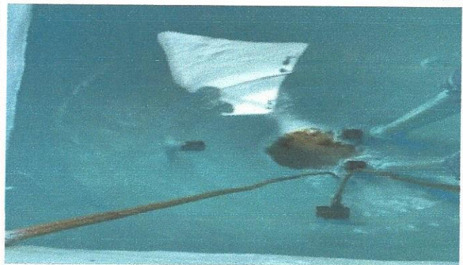
Walnut Lift Station after Alumiliner and Raven 405 Epoxy
