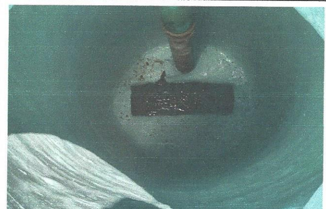
Walnut Lift Station after Alumiliner and Raven 405 Epoxy
